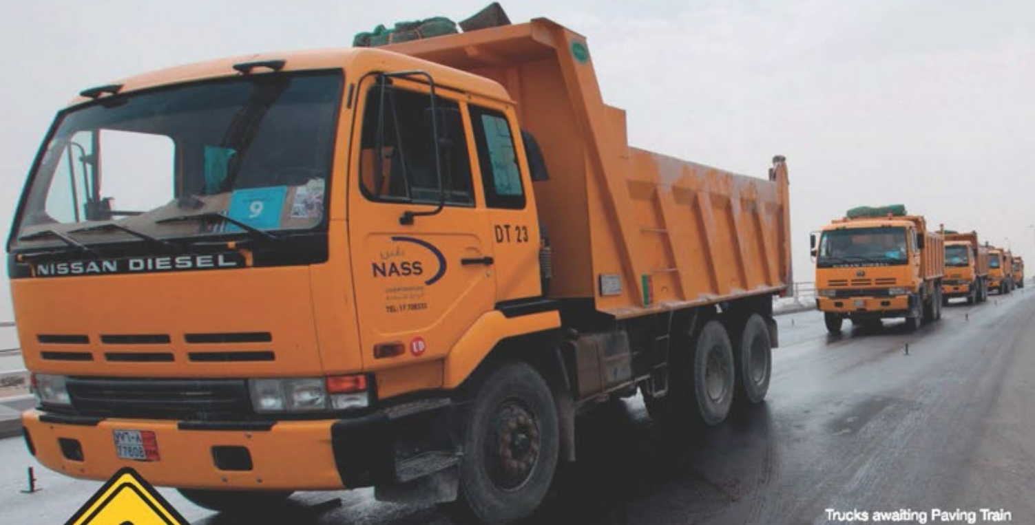
Trucks awaiting Paving Train
