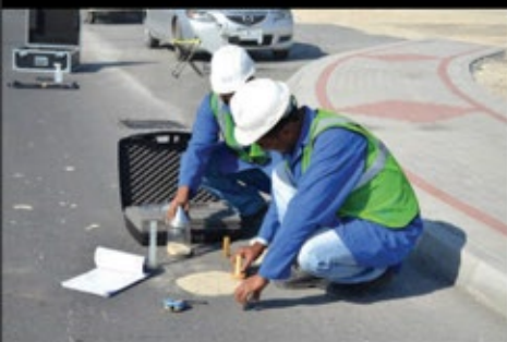
Sand Patch Test
